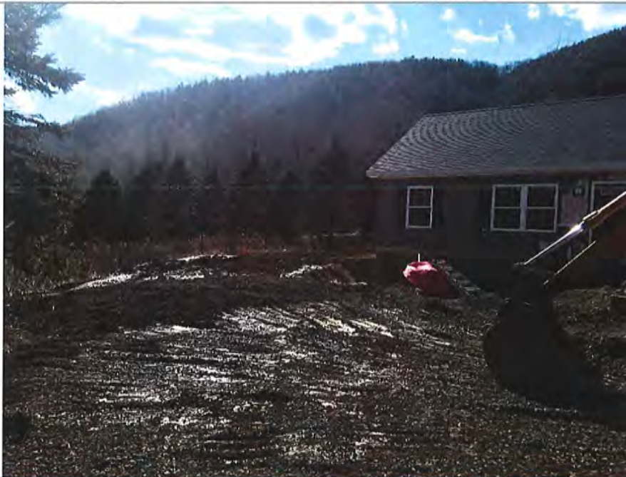
Site visit to 111 Patchen Court 2/27/18 showing partially built home and extent of disturbed soil.
